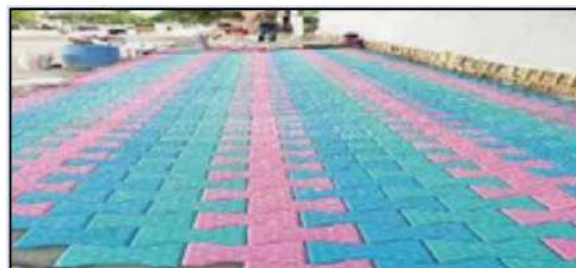
Figure 9.12 Pavement constructed using recycled plastic tiles (MoHUA, 2019)
